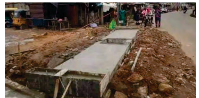
Picture of one of the ongoing culverts construction
